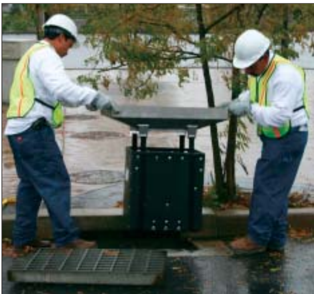
The lightweight Drop In series of the Ultra Urban Filter is quickly and easily installed.
